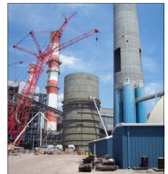
The scrubber at Wateree is under construction.
