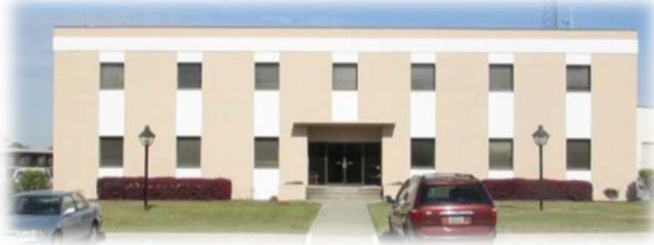
Former Gas Operations Center
