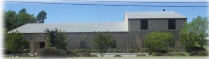
Former Gas Measurements Bldg.
